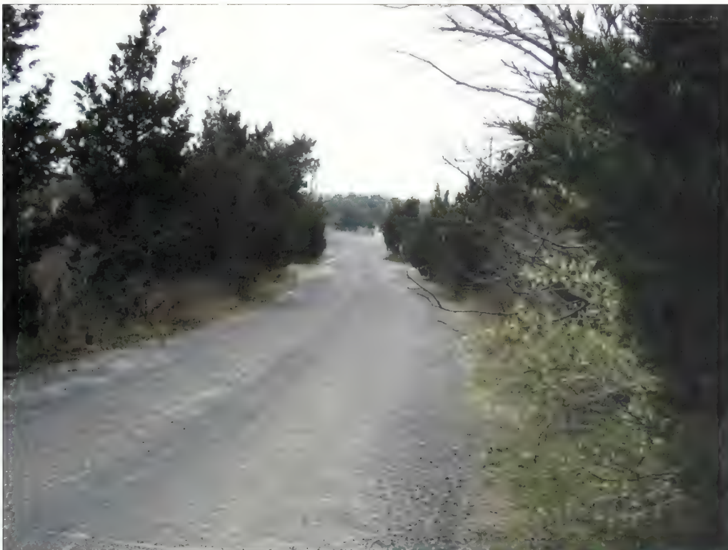
Figure 5.113. View looking northwest toward Ready Barracks, NIKE launch site. This photograph shows the vehicular route has become overgrown and feels like a tight corridor in contrast to the open, low-growing vegetation in the historic image. The overgrown vegetation limits vehicular sight-distances and may put pedestrians at risk if park visitors use this route as a walkway during the hours of active maintenance operations (Olmsted Center, April 2008).
